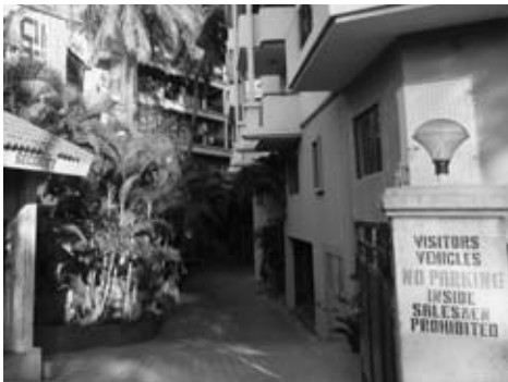
Entrance of apartment building in Richmond Town
